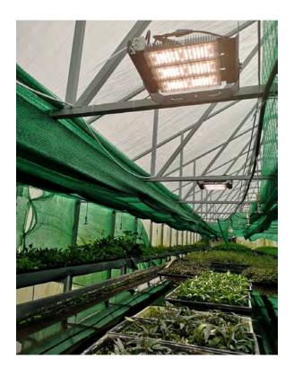
These lights have a special spectrum that radiates extra energy in the blue and red range, but is cold white to the eye looking LED is a good choice for both plants and the human eye to work with. The traditional blue + red LED combination based on new research is no longer worth using because the plants have the rest they also need color for optimal growth.
